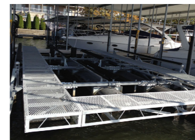
Surface platform walkway
