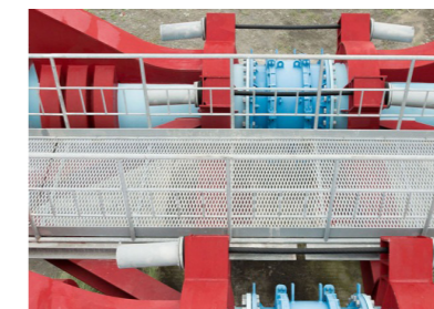
Overhead pipe walkway
