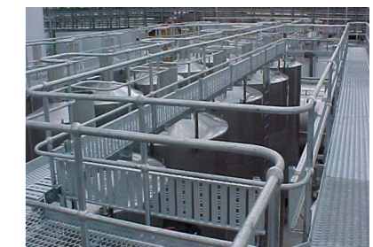
Industrial platform walkway
